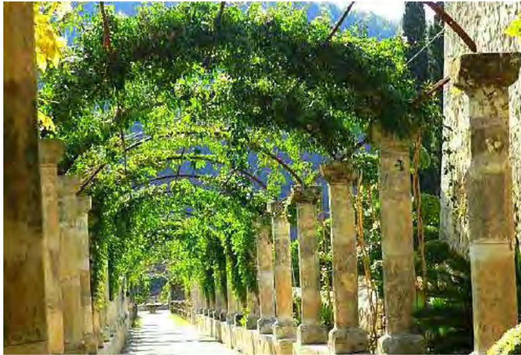
STEEL FRAMEWORK & STONE COLUMNS TO GAZEBO
