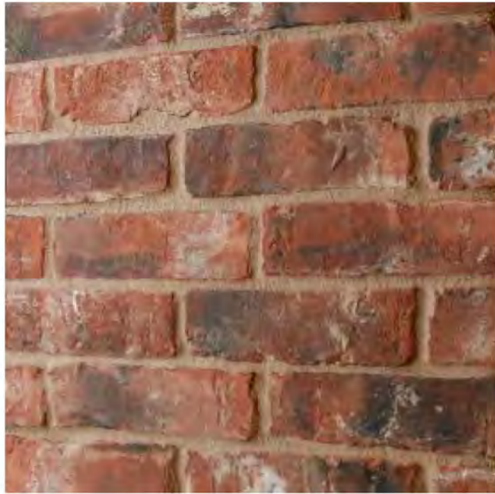
RECYCLED BRICK WALLS
