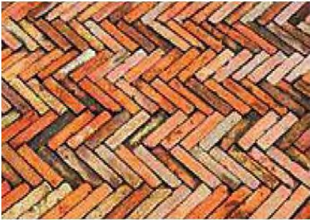
RECYCLED BRICK PAVERS
